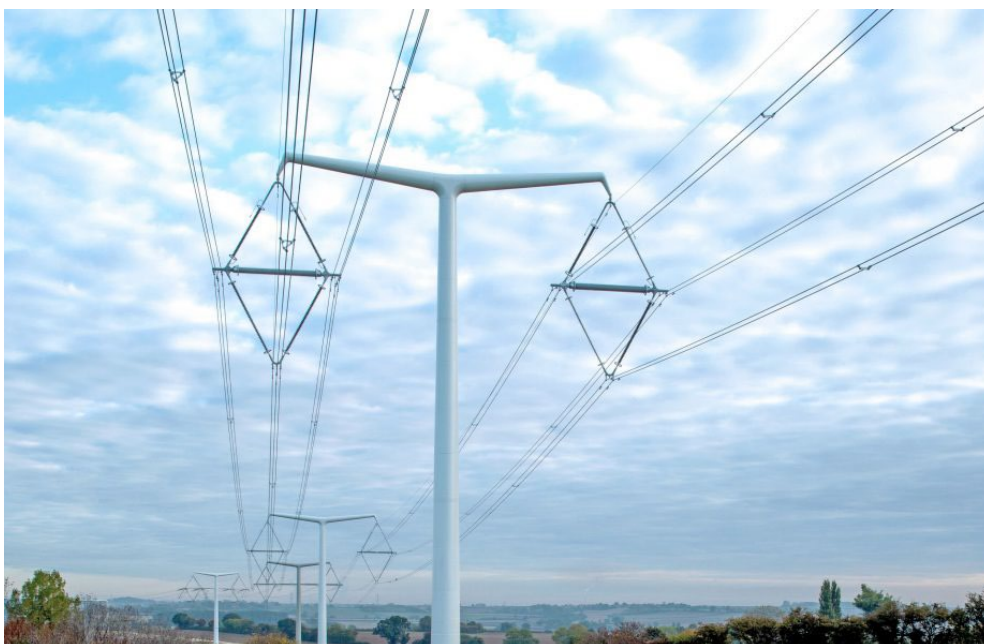
Image 1.3 Typical suspension T-ylon
